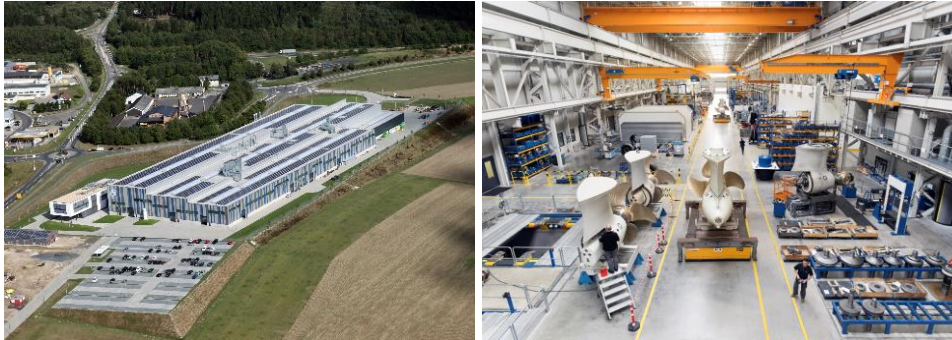
Bilder 6+7 (SCHOTTEL_100 Jahre_06.jpg), (SCHOTTEL_100 Jahre_07.jpg) Aerial view and interior view of production site in Dörth
