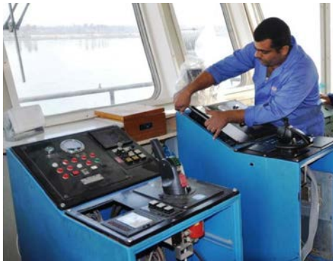
Customized upgrade of control system
