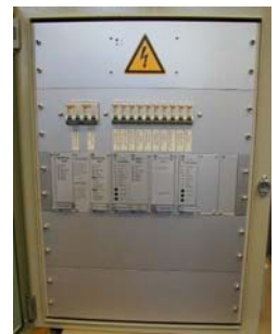
Switch box with steering cards
