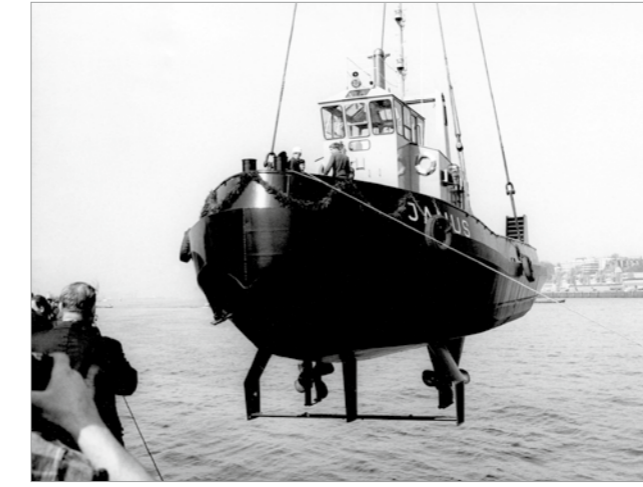
The Janus enables SCHOTTEL to enter the tug market at the end of the 1960s.
