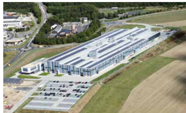
The total area in Dörth covers 9 hectares. The production halls, which are arranged to suit the material flow, measure up to 280 metres in length.
