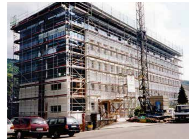
The addition of another floor to the existing administration building at the turn of the millennium addresses the demand for more space in administration as well.
